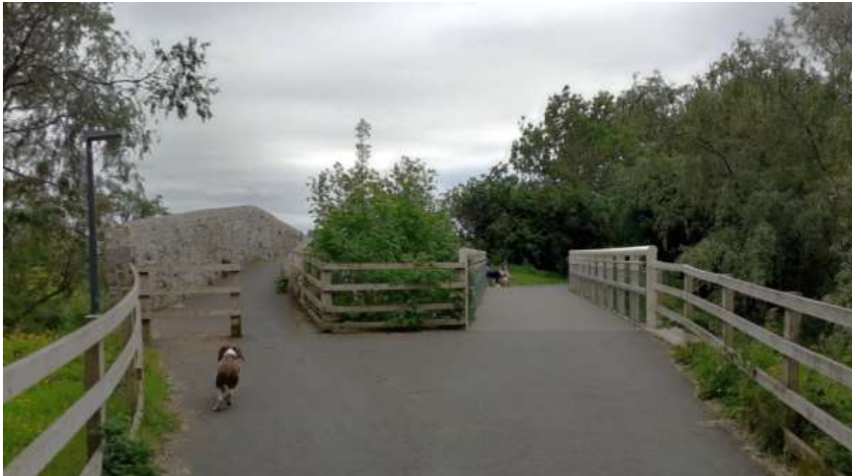
Figure 6-1: Existing Bridge at River Groody
