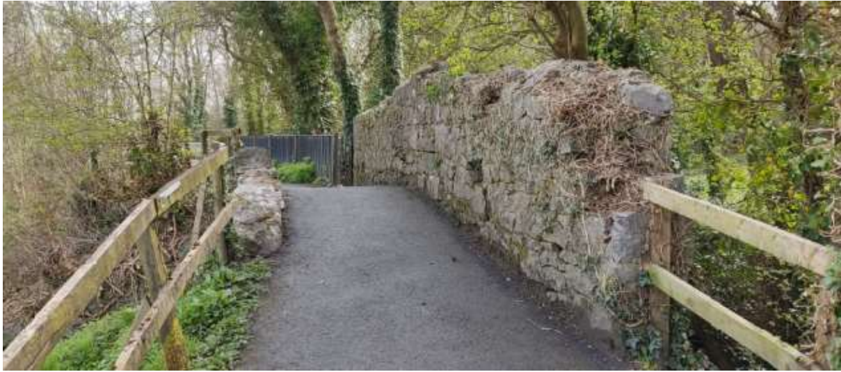
Figure 6-16: View of Bridge 2 from the exiting paved path
