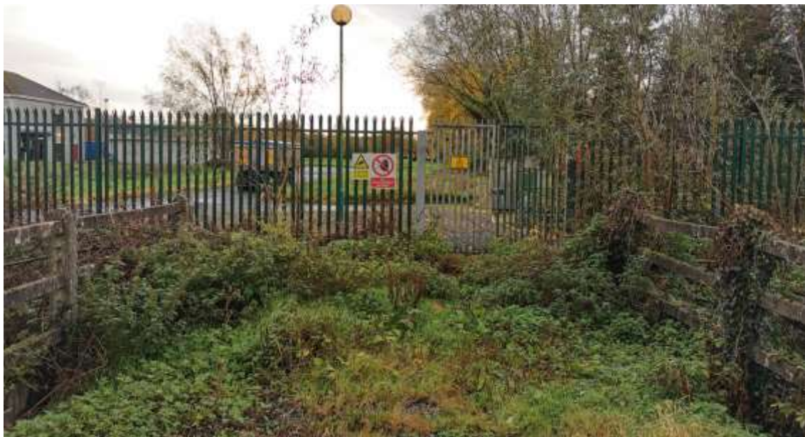
Figure 6-13: View south to the northern access gate of Castletroy Wastewater Treatment Plant
