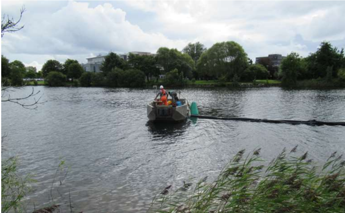
Figure 6-85: Installation of a silt curtain in the River Corrib, Co. Galway
