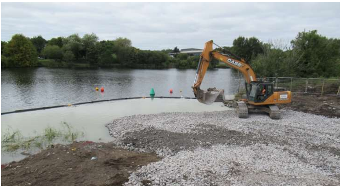
Figure 6-86: Silt curtain retaining contaminated water during advanced works for sheet piling
