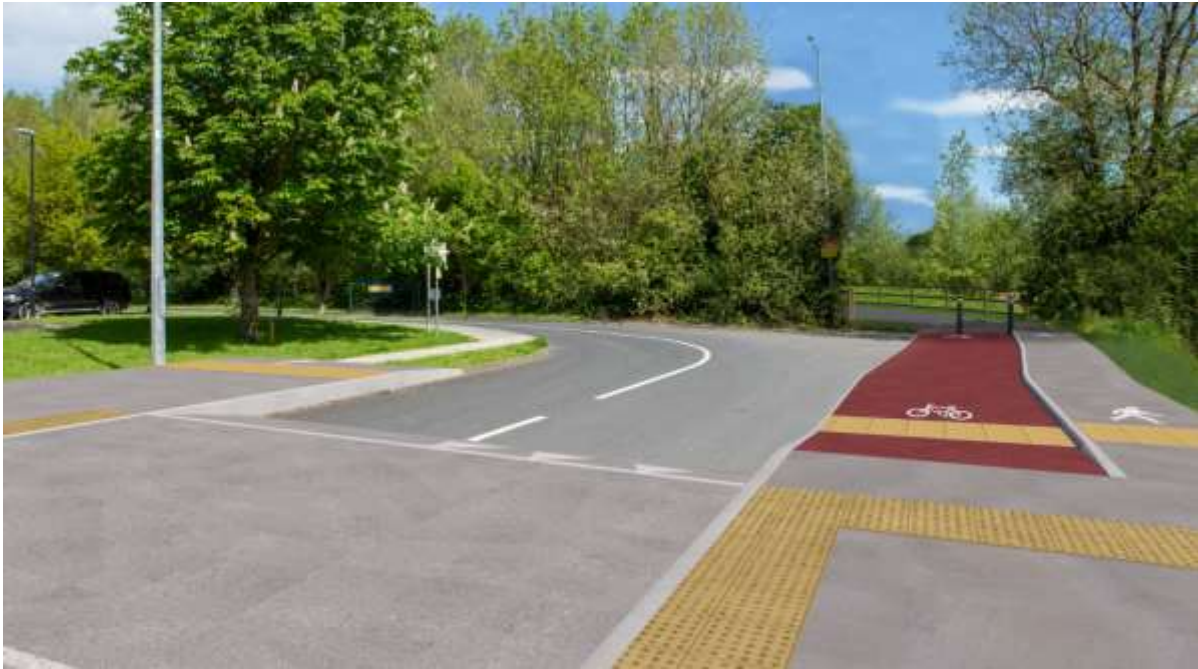
Figure 6-117: Proposed cycle lanes and footpath on McLaughlan Road where it joins the shared path
