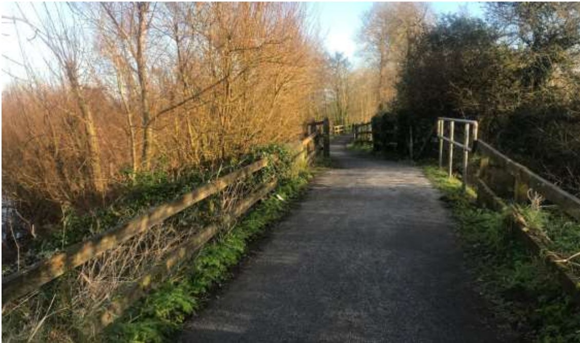
Figure 6-10: Existing Bridge No 1
