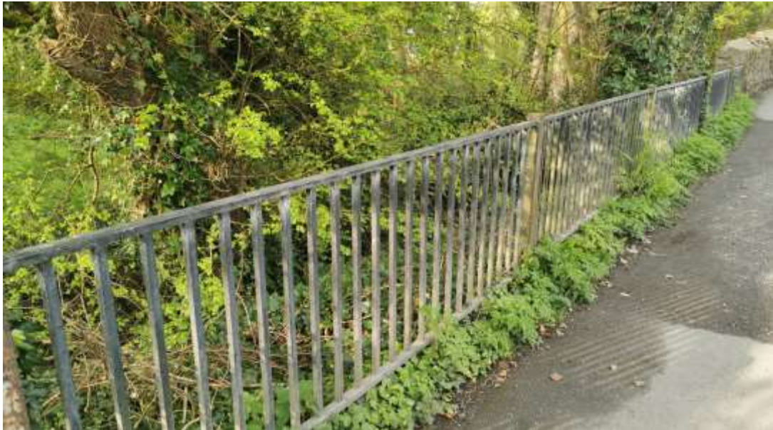
Figure 6-19: Existing railing between Bridge 2 and Bridge 3
