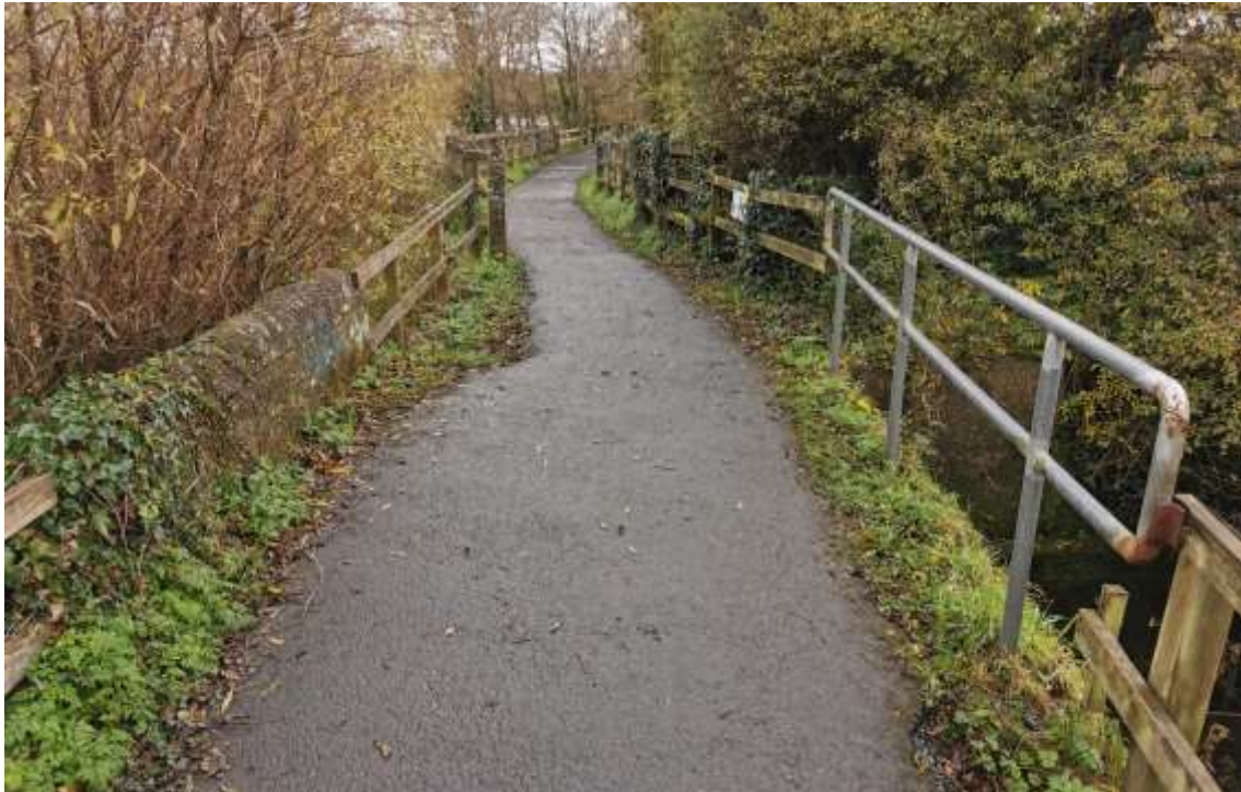
Figure 6-11: Existing bridge over land drain (Bridge 1)
