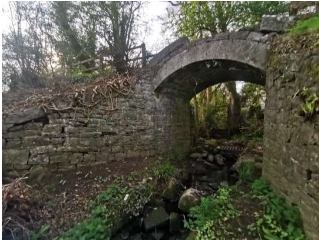
Figure 6-17: View of Bridge 2 from bank of drain
