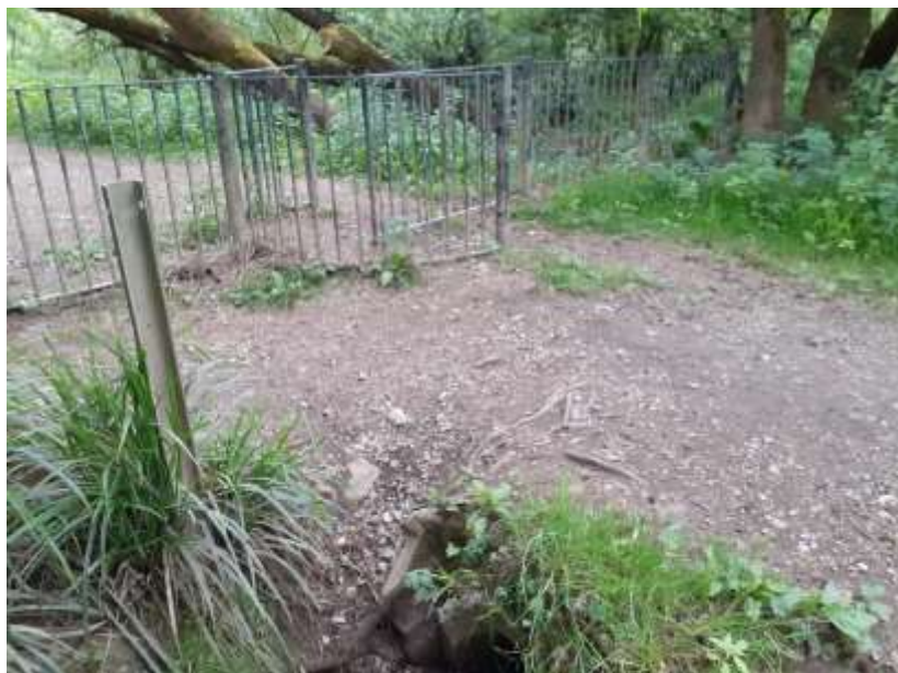
Figure 6-54: Existing gate and culvert at the land boundary between UL and the IDA
