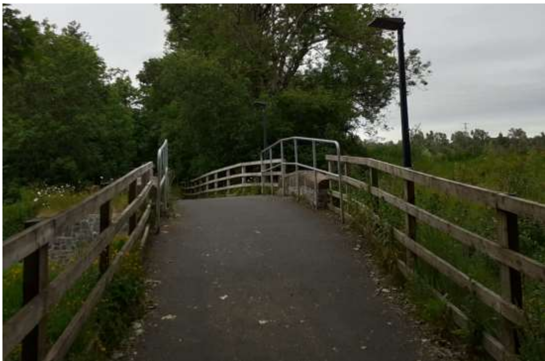
Figure 6-3: Existing bridge at CH400
