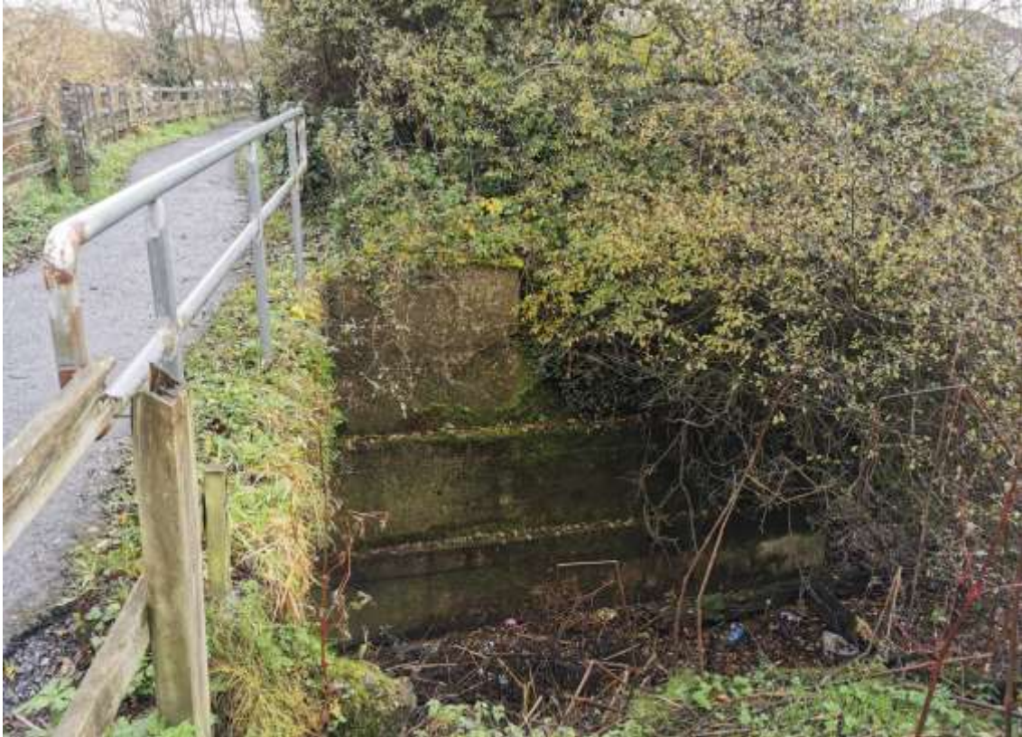
Figure 6-12: Existing abutment wall (proposed to be decommissioned)
