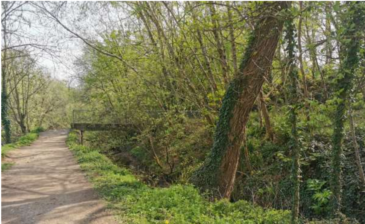
Figure 6-48: Existing concrete bridge at mouth of Plassey mill race (to be retained)
