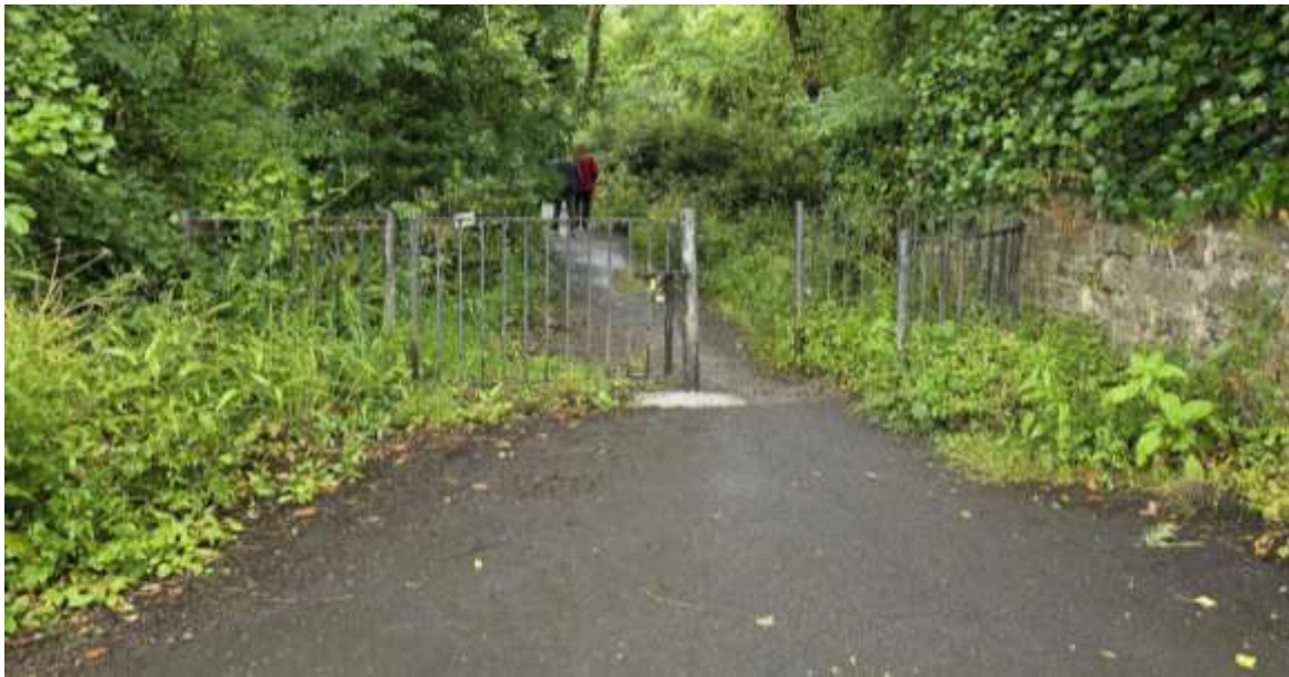
Figure 6-25: Existing gate on path at Plassey Mills (1 of 2)
