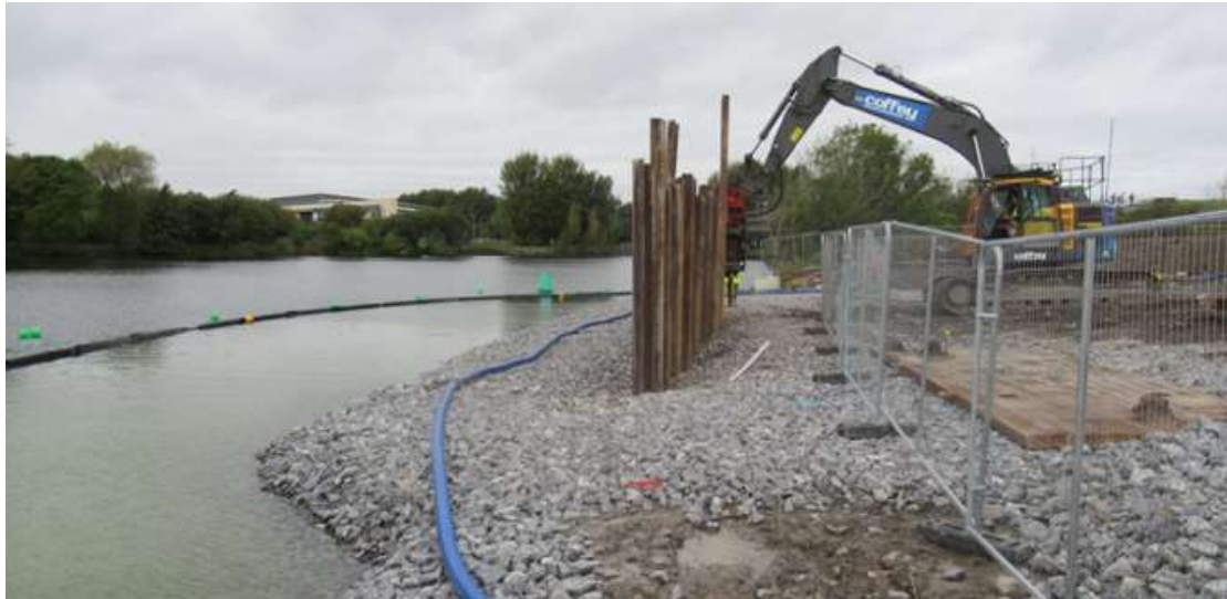
Figure 6-87: Example of sheet piling along the bank of the River Corrib
