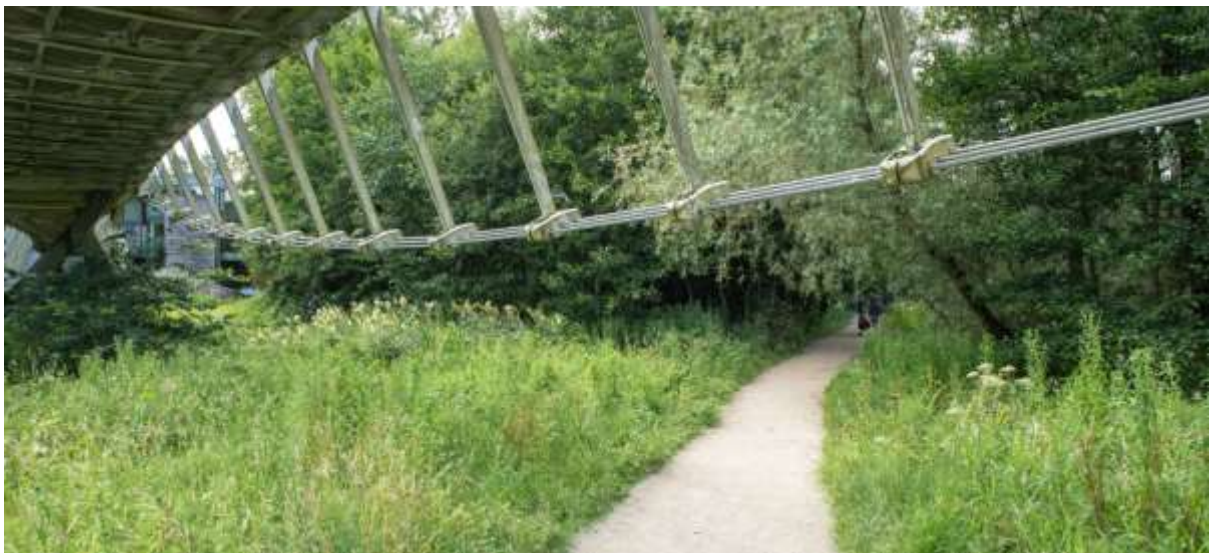
Figure 6-43: Existing gravel path under the Living Bridge
