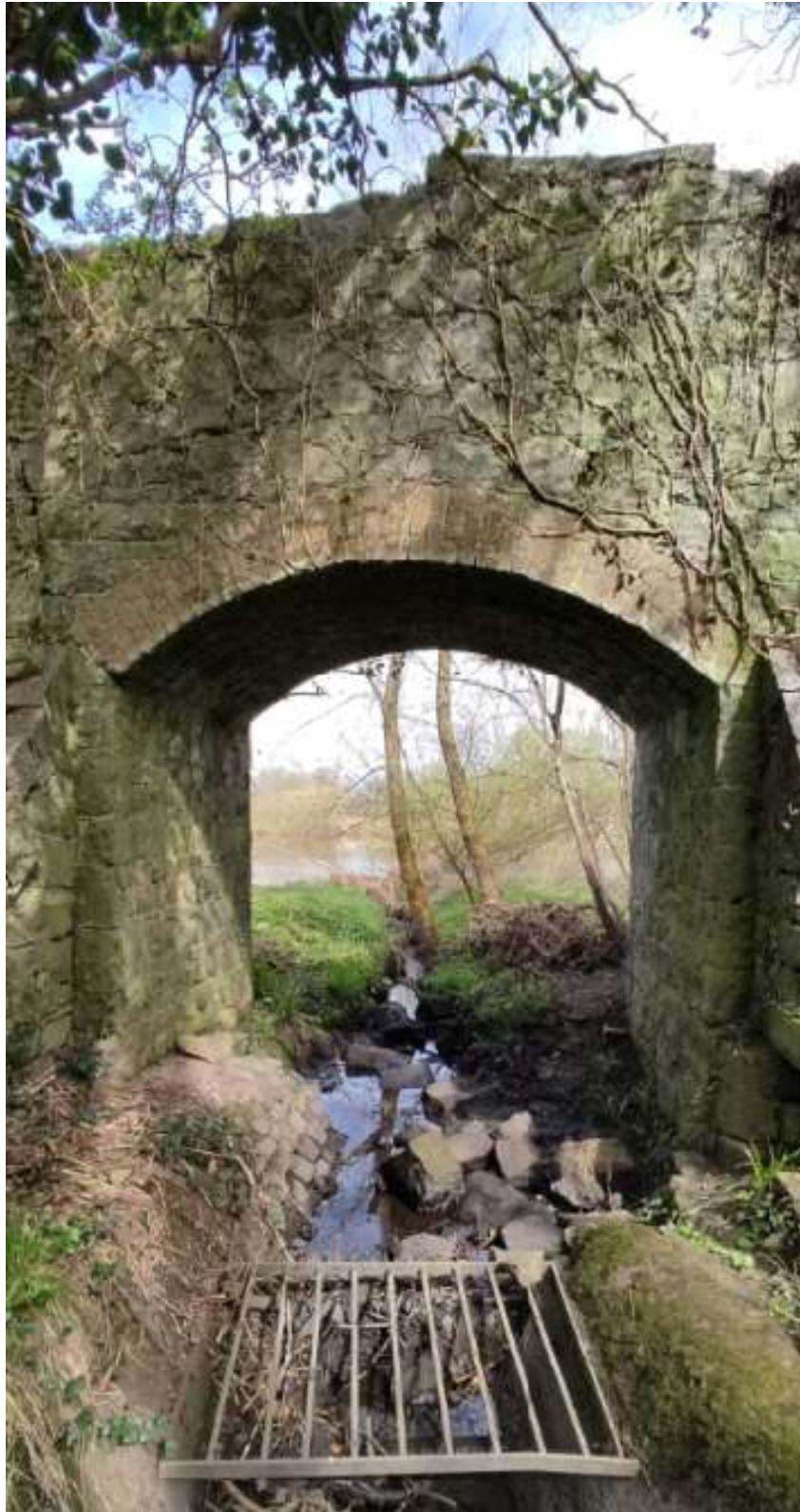
Figure 6-18: View under Bridge 2 facing north to the River Shannon
