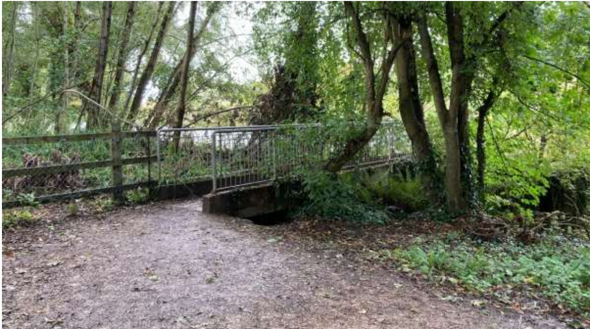
Figure 6-50: Existing concrete bridge at mouth of Plassey mill race looking northeast
