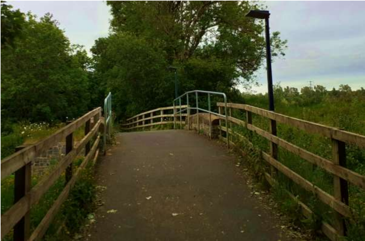
Figure 6-78: Existing bridge at CH400
