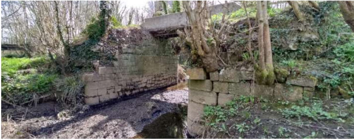
Figure 6-21: Shallow water level in Plassey Mill Race and existing abutments of Bridge 3
