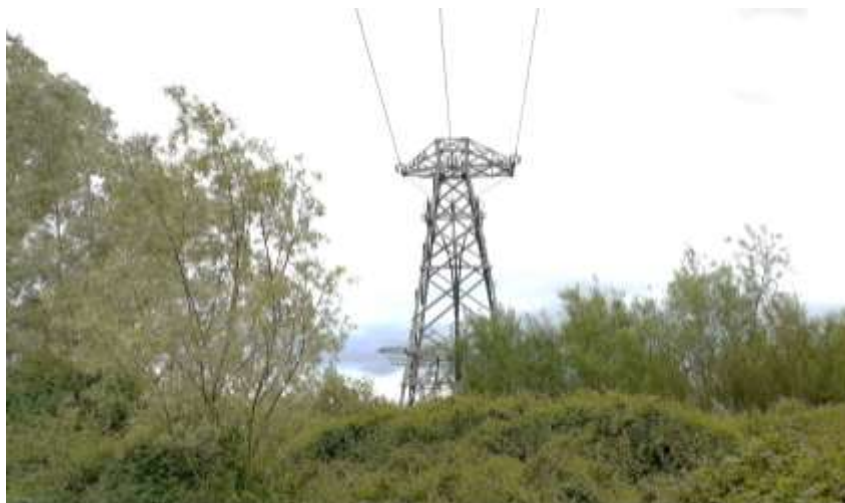
Figure 6-61: Overhead ESB utilities
