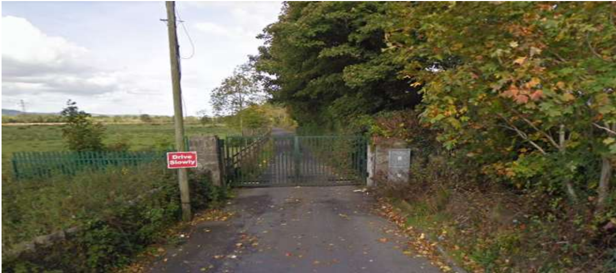
Figure 7-11: Access to Section 1 from the entrance road to the Castletroy WwTP
