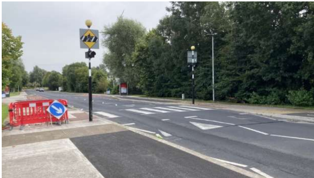
Figure 6-120: The existing Zebra crossing on Plassey Park Road proposed to be converted to a Toucan crossing
